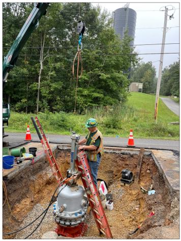
Mueller A.W.W.A Standard Gate Valves). The valve may then be operated like any standard gate valve. PermaSeal™ Insertion Valves can be furnished with a handwheel and post indicator plates when specified. All PermaSeal Insertion valves have a full-size water way. MUELLER PermaSeal™ Resilient Wedge Insertion Gate Valves meet or exceed all pertinent requirements of ANSI/AWWA C515-15 gate valve standard. They are ANSI/NSF 61 & 372 certified for drinking water components.
